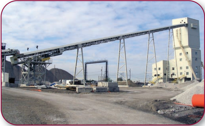
42" x 326' Stationary Feed Conveyor
